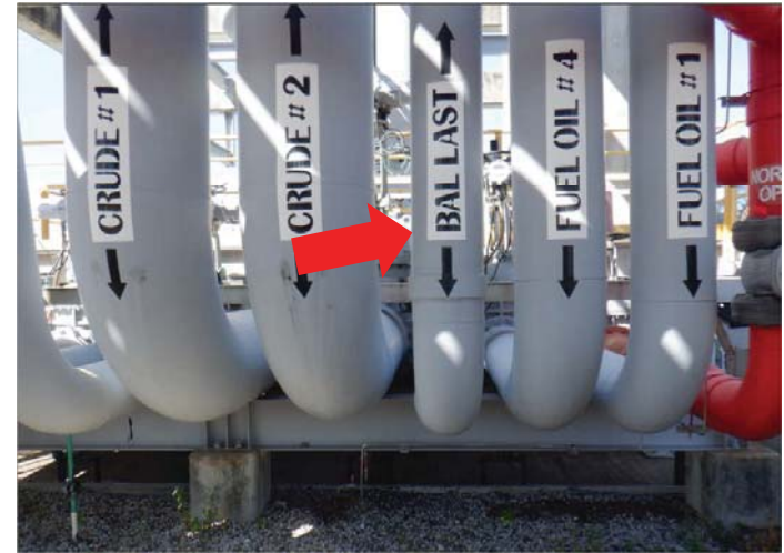
Photo1: 12" Ballast line from Marine Product Pier to shoreline.
