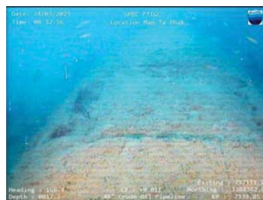
Typical Field Joint
