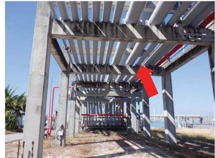
Photo1: 12" Ballast line from Marine Product Pier to shoreline.
